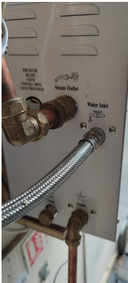
Recommended: Use flexible pipe for water inlet.
